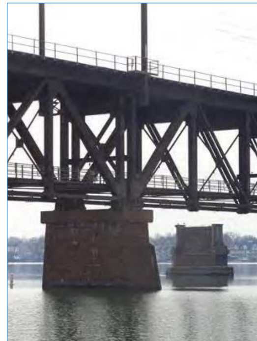
Existing Susquehanna River Rail Bridge
