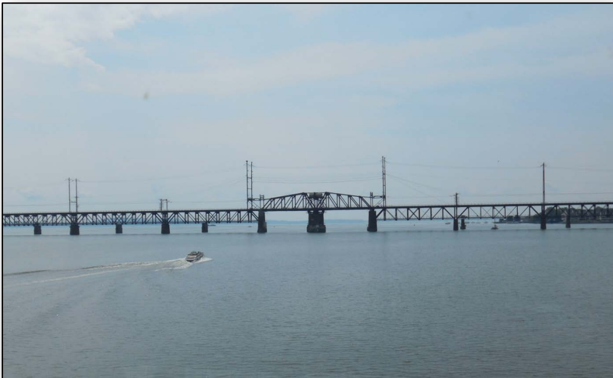
Photo 1: Amtrak Movable Bridge over Susquehanna River, Upstream (West) Fascia
