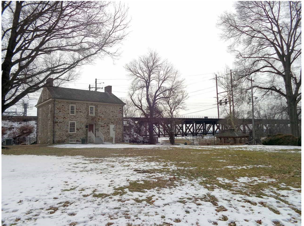
View looking southwest of the north façade of Rodgers Tavern and the Susquehanna River Rail Bridge abutment and embankment to the north. 13
