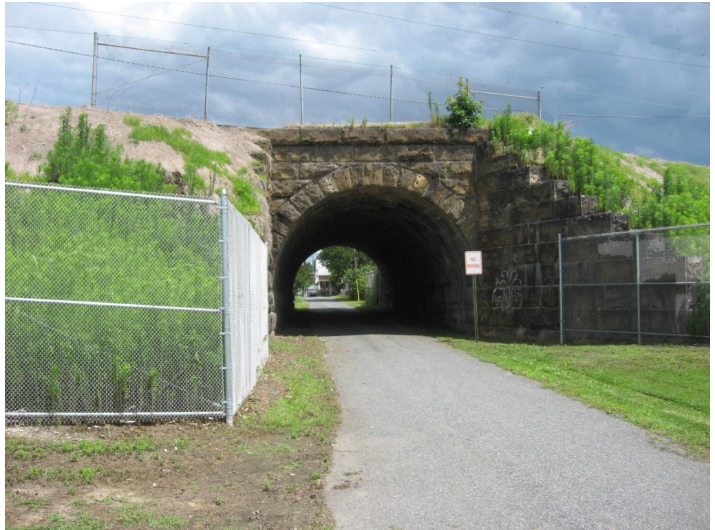
View looking north at the Centennial Lane Undergrade Bridge (MP 60.61), one of nine undergrade bridges considered historically significant in relation to the Susquehanna River Rail Bridge. 3
