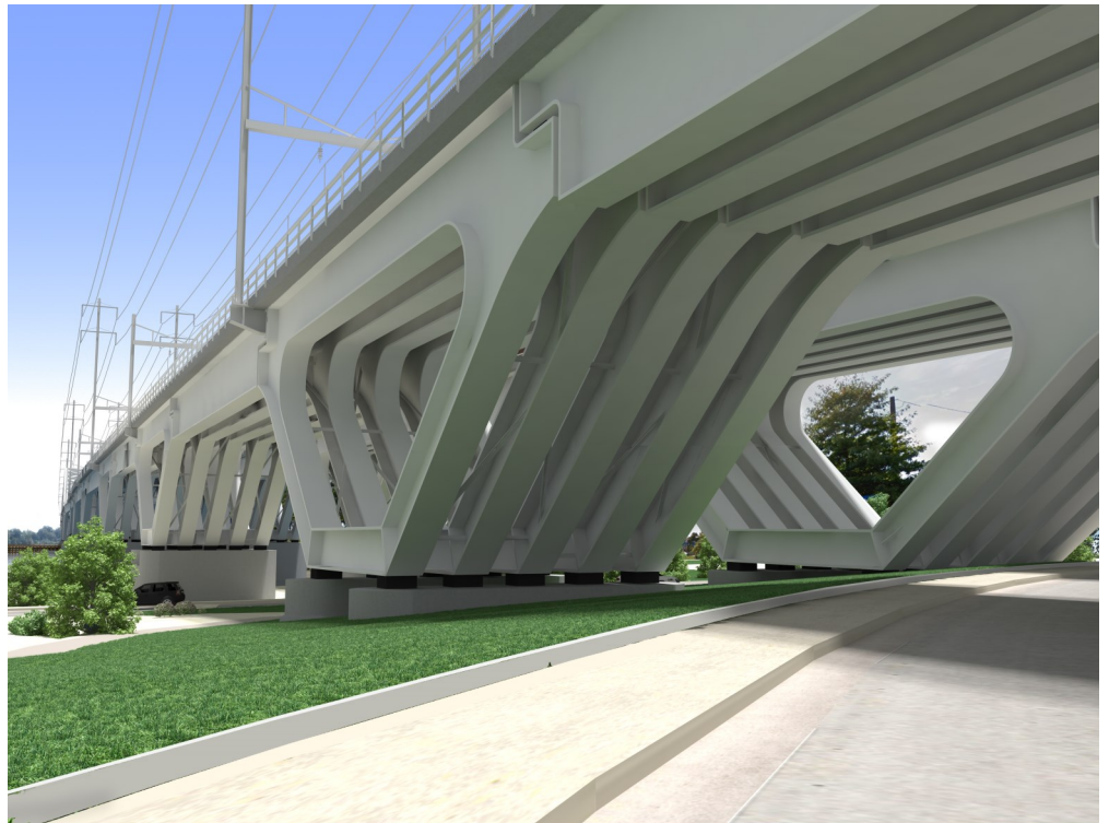
Rendering of the piers for the Delta Frame approach. 33
