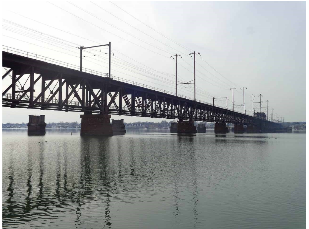
View looking west at the Susquehanna River Rail Bridge from the Perryville waterfront. 2
