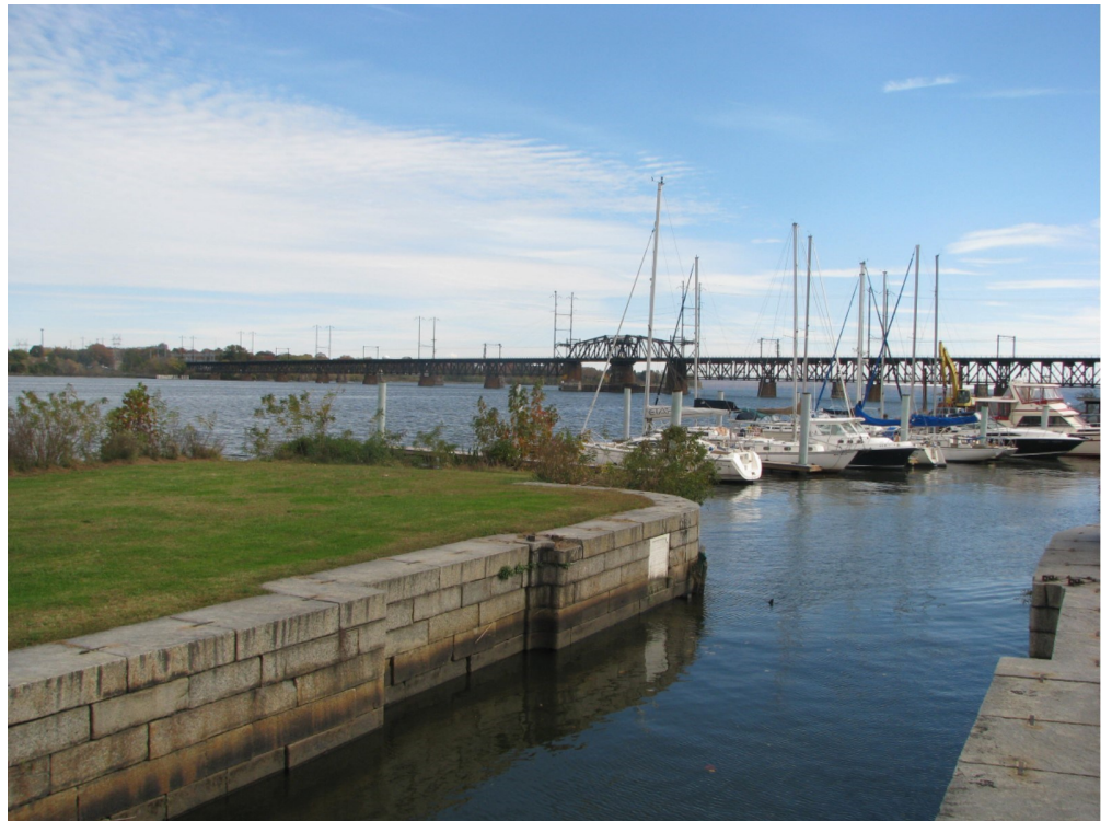
View looking south from the Southern Terminus, Susquehanna and Tidewater Canal - South Lock #1 and Toll House towards the Susquehanna River Rail Bridge in the distance. 12
