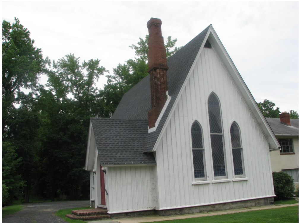
View looking southeast towards the NEC from the Perryville Presbyterian Church. 18
