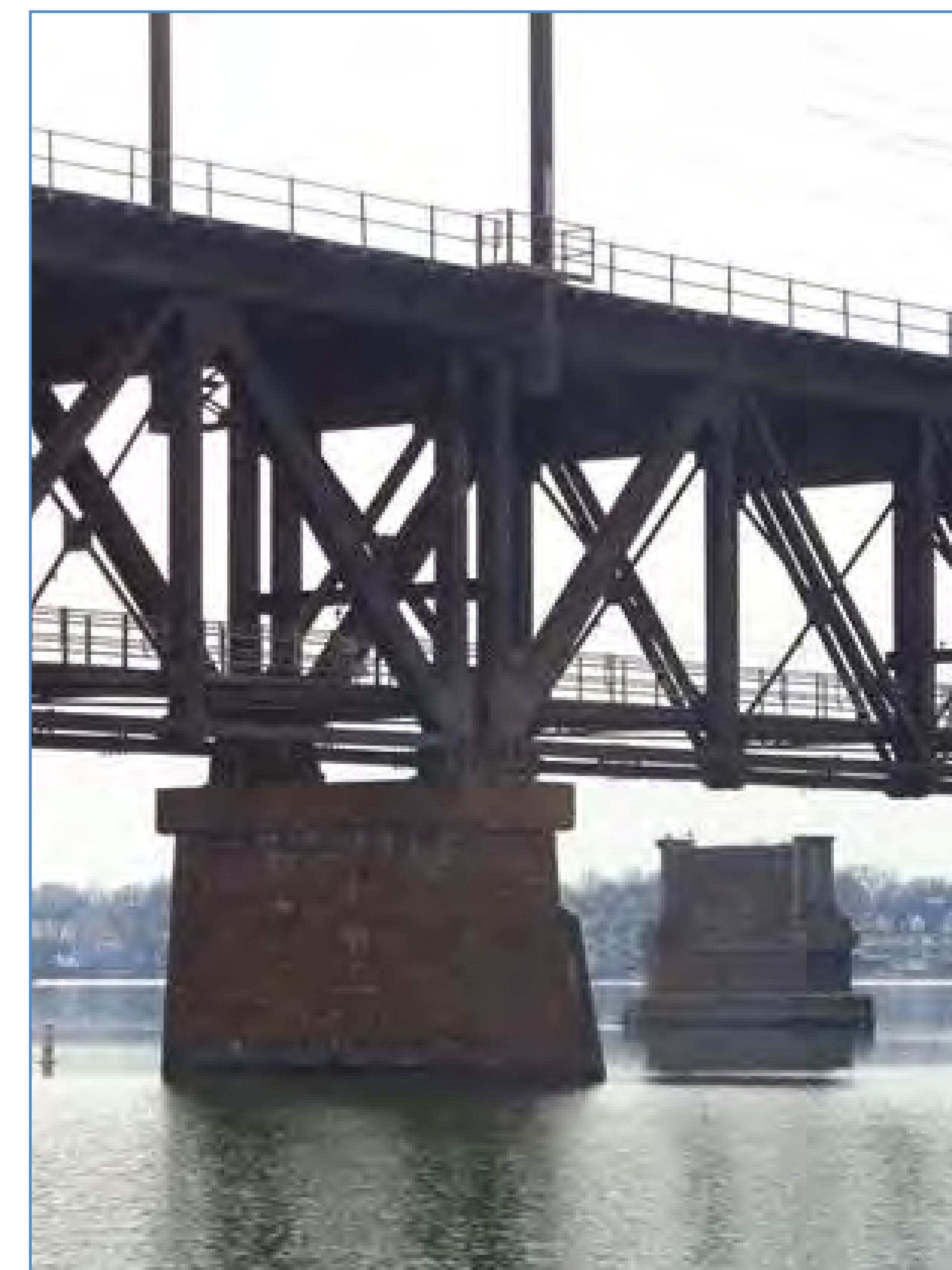
Existing Susquehanna River Rail Bridge
