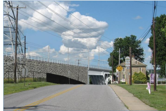
Retaining Wall with Delta Frame Design
