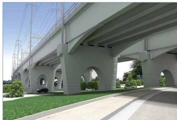
Key Hole Pier Design
