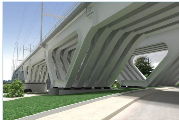
Delta Frame Pier Design
