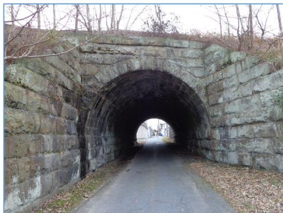
Potentially Historic Undergrade Culvert (Centennial Lane)
