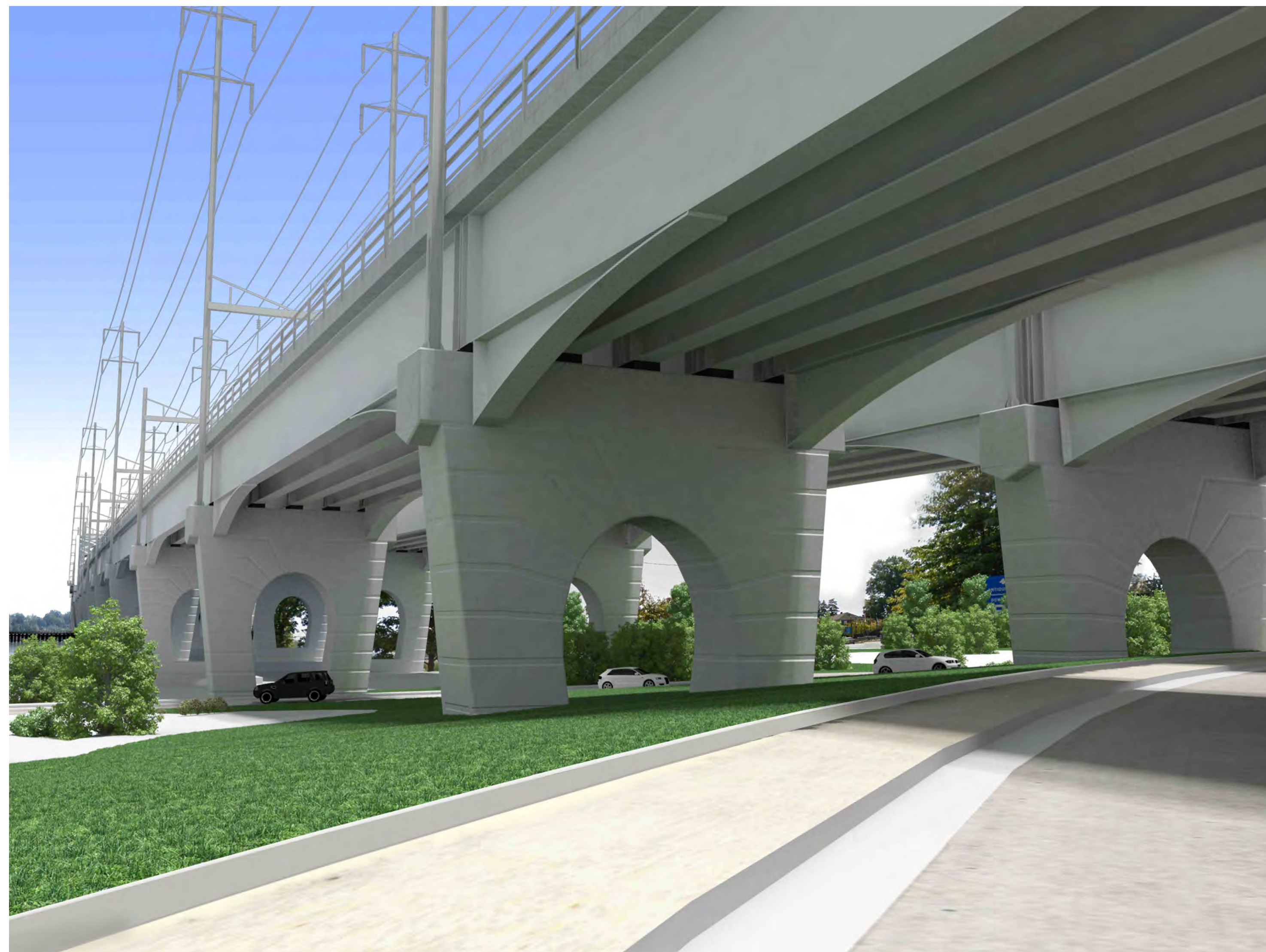
Key Hole Pier Design
